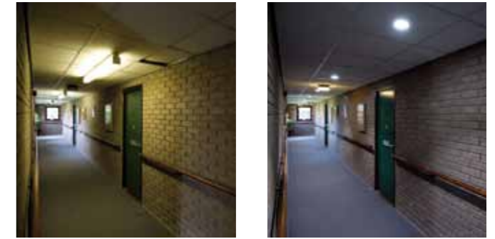
Pre-installation and post-installation
