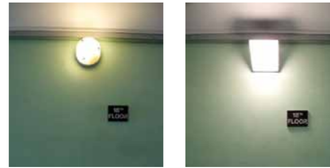
Pre-installation and post-installation
